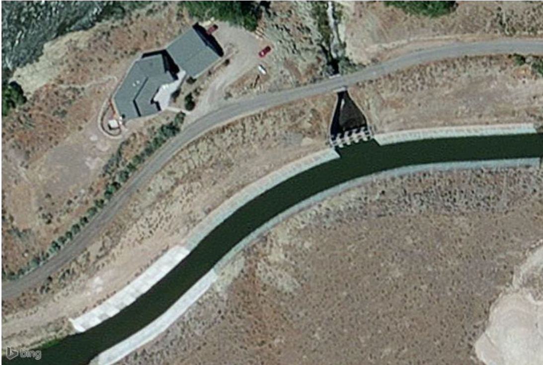
Figure 9.2-11. Segment of Truckee-Irrigation District Canal
