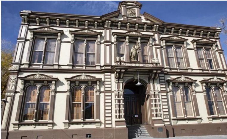
Figure 16: Built in 1875, the Storey County Courthouse still facilitates most county offices as well as the District Court. Although nostalgic, over $2 million is needed to bring the building to current codes and perform repairs, and the county has outgrown the constricted spaces of the building. The building should be considered for future official use; however, additional facilities are being considered to relieve pressure from this historic building.
