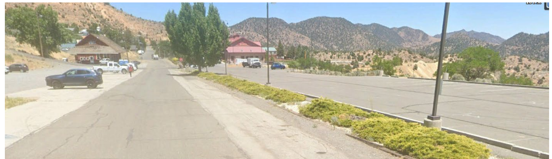
View of the property from E Street looking north, VC Freight Depot is on the left, Silverland Inn on the right.
